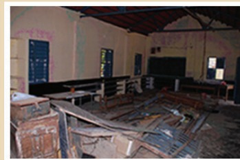
TNF Pilot Project - Before: Unused panchayat school building
